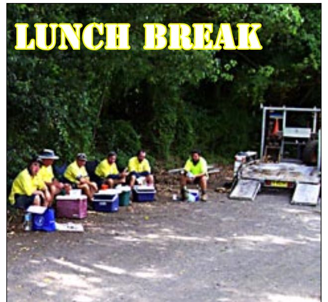
Lismore Council's bridge working team taking a lunch break at the Bush Theatre carpark while doing repairs to Cullen Bridge.
