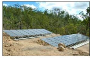
Company, its biggest installation to date. The system consists of a 12 KVA inverter, 90 x 130 watt solar panels delivering 120 volts DC into 60 x 2 volt 1660 amph batteries. It produces 11.7 kilowatts, and will save 26,000 litres of diesel, or 78 tonnes of CO2 emissions.
