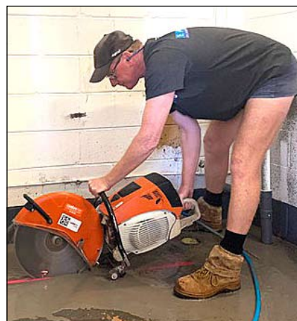
Plumber Rob Gall preparing to install new drainage and water lines prior to the tiling of the toilet block.
